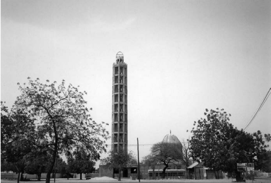
Figure 7.1. A new grand mosque under construction in Darou Marnane, a satellite town of Darou Mousty. Photo by author, 1997.
